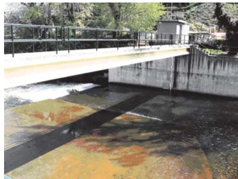
Gauging station of the Iregua river in Islallana (La Rioja)
